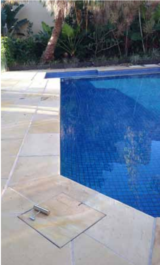
Central edge Keyway: Easily cut with 4 inch grinder.
